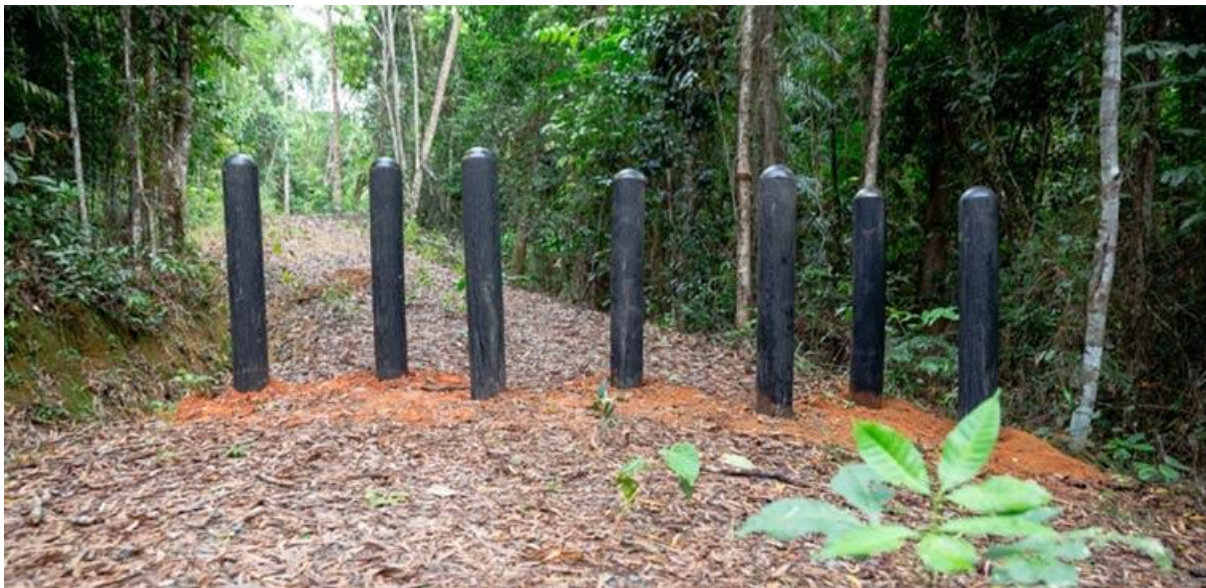
Figure 3 Bollards made from recycled old tyres in the Daintree Rainforest (Bridgestone Tyres, 2017)
